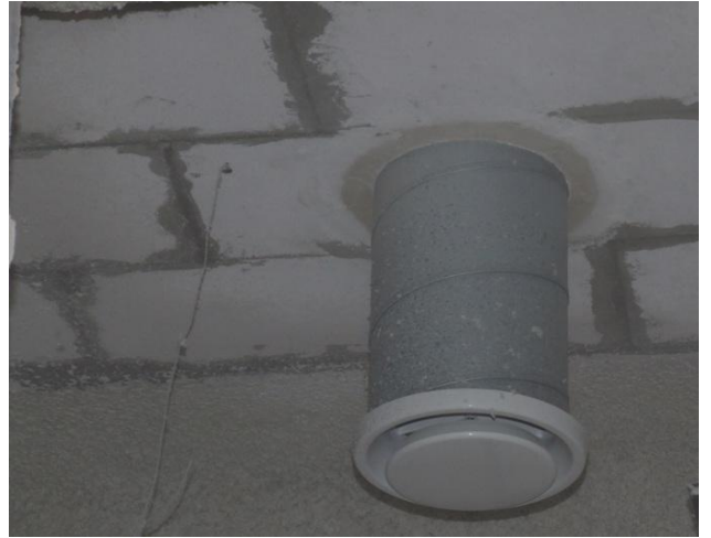
Exposed face of the test specimen before the test commencement
