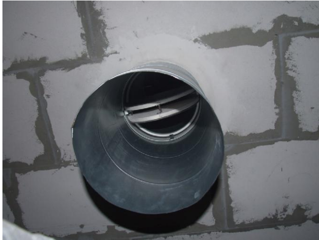
Exposed face of the test specimen during the test preparation process
